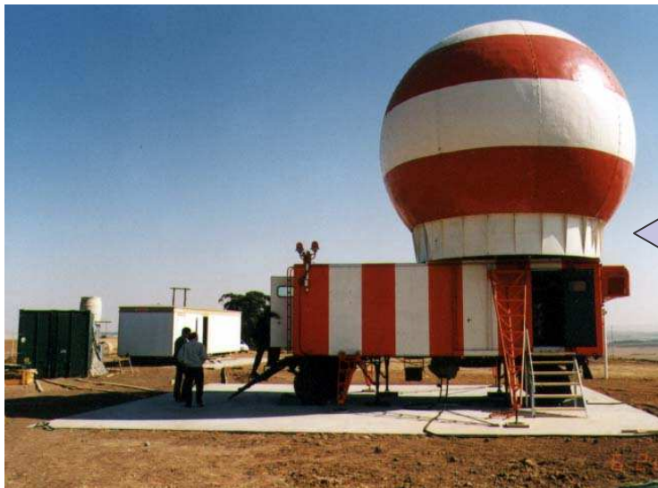
Radar Assembly completed (July 1994)
